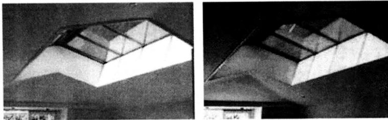
**Figure 3** Examples of color-reversibly changeable electrochromic glass for skylight applications in building [4]
